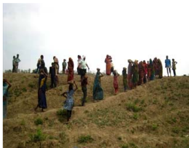
Repair of earthen check dam through Shramdan (worth Rs. 57,000), Gopalpura, Chattarpur
