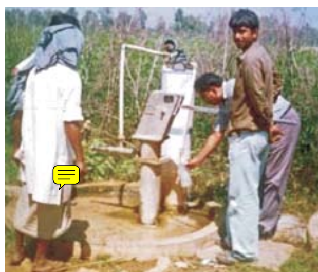
Defunct defluoridation unit attached to handpump in palamau, Jharkand
