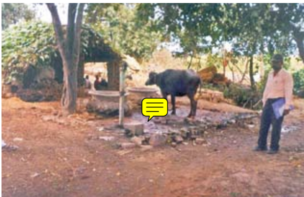
No apron area and animal interference to the source (Handpump of Ravendra Prasad, village Paharpur)
