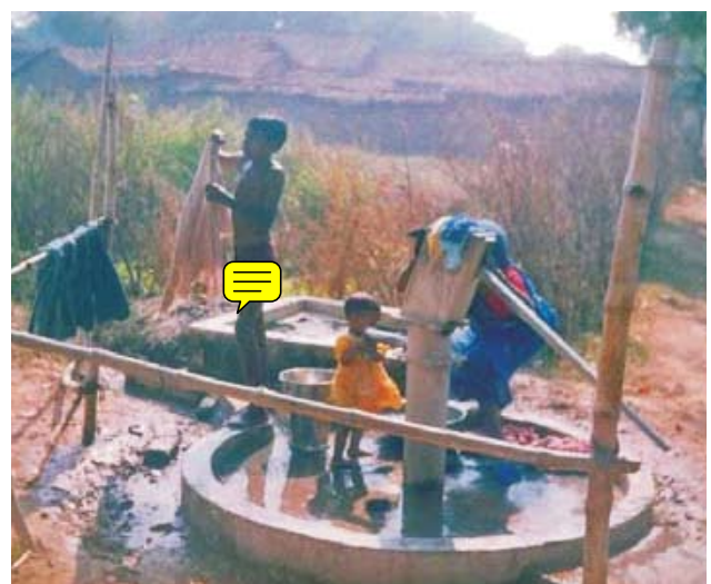
Prevention of animal interference but spreading of water around the source (Handpump near Sharda Prasad Yadav's house, village Tulsi Purwa, U.P.)
