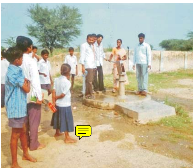
Spreading of water and no drainage around the source (Handpump at Thimma Reddy Nagar, Mehboobnagar)
