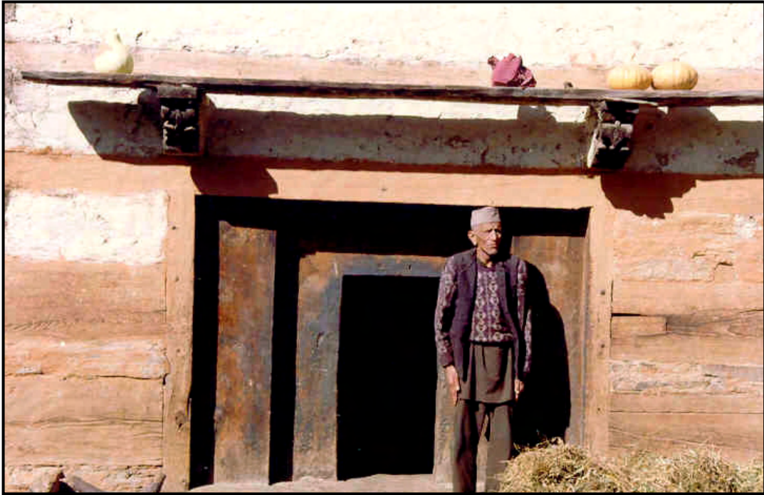
Small openings are an important quake-resistant feature
