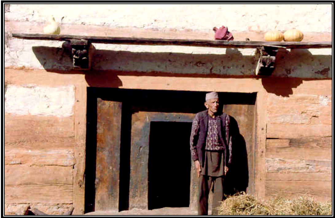
Small openings are an important quake-resistant feature
