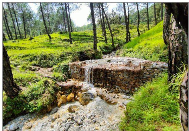
Gabion Check Dams (GCD) Construction of for reducing the velocity of water of
